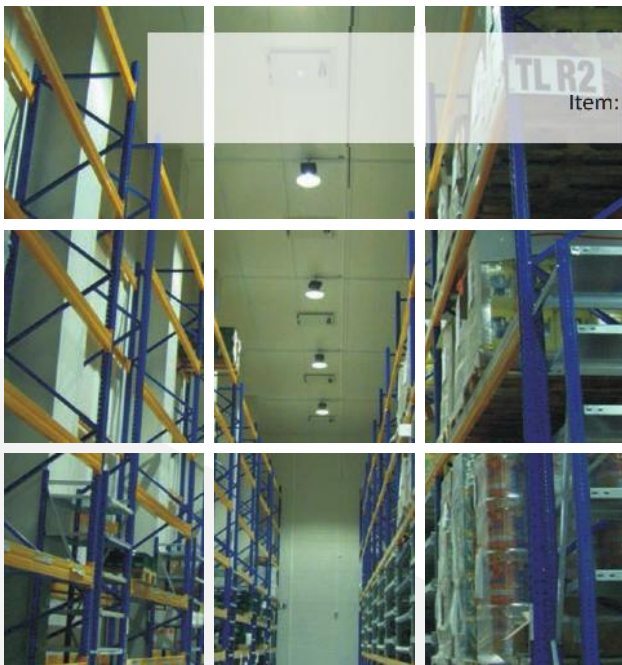
Location: ILPEA Industries, Italy Item: Lumedgo 150W LED high bay light / LMHB-150A / retrofit 400W HID
